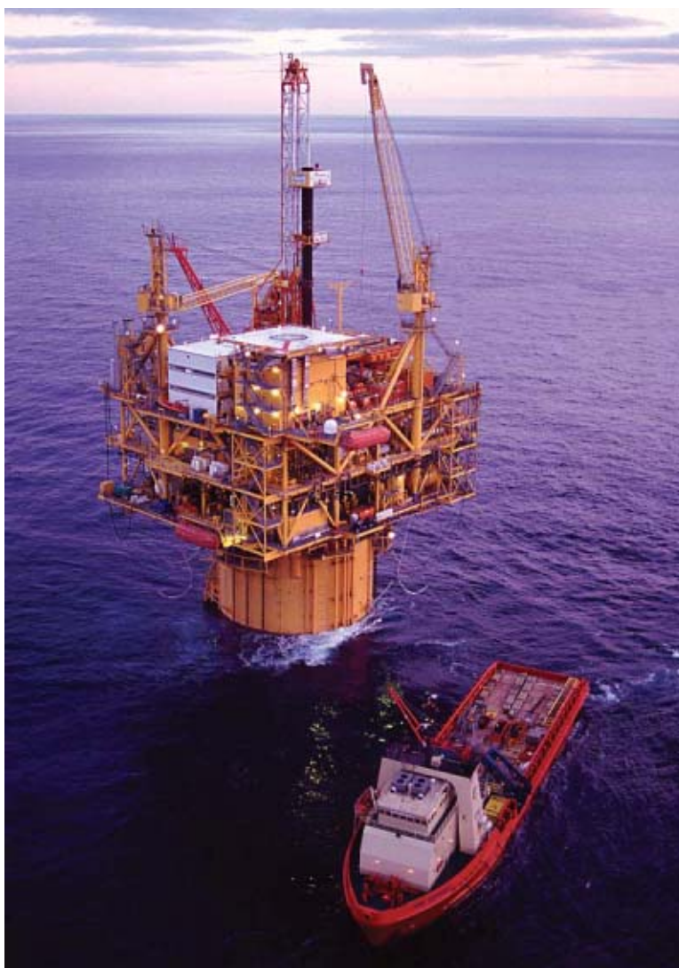
Devil's Tower truss spar in the ultradeepwater Gulf of Mexico has capacity for 60,000 b/d of oil and 110 MMcfd of natural gas. Photo courtesy of Dominion Exploration & Production.
